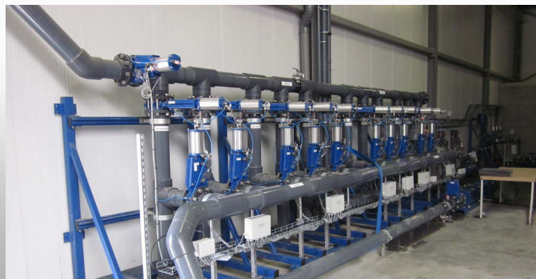
Due to the number of tanks, the demands on the central pump block are high.
