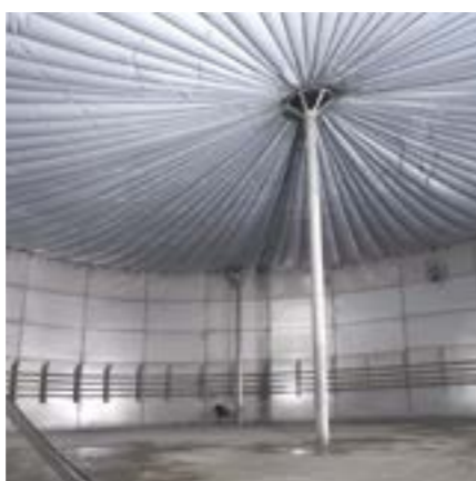
Digester, interior view
