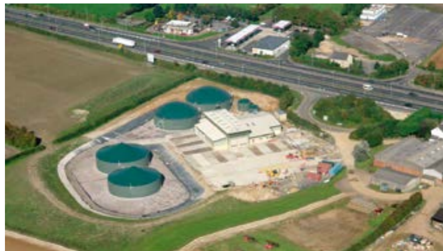
In the United Kingdom, the energy recovery of organic residues by digestion is much more common than in Germany. Here is an aerial view of a WELTEC plant in Kettering (England).
