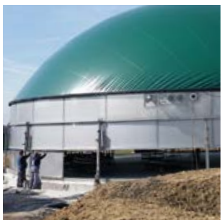
Setting of tank in segments
