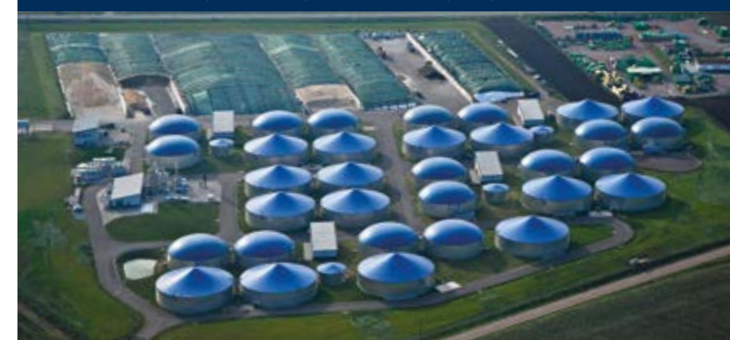
Bottom: The biomethane refinery Könnern (Saxony-Anhalt) is one of the largest biogas plants in the world.
