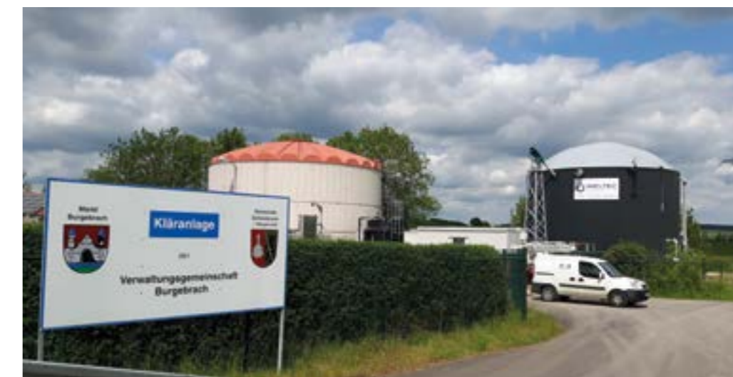
The stainless steel fermenter (right) in Burgebrach now ensures efficient digestion and stabilization of the sewage sludge.
