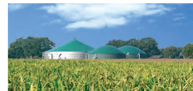
Agricultural Biogas in Oldenburg Münsterland (Northern Germany)
