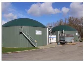
To maintain an optimum stock level, an underground pre-storage tank is located before the two 2,625-m³ stainless-steel digesters.
