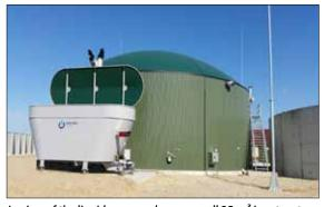
In view of the liquid manure share, a small 35-m<sup>3</sup> input system is sufficient for transferring the solid substances, such as maize silage.
